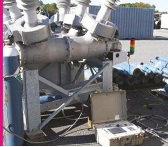
Smartfill CTU is a unique SF6 “live top up” device designed for managing SF6 leaks to ensure critical assets remain operational.
